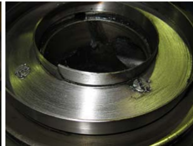
Baffle plate fractured
