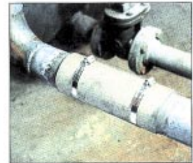
REPAIR CORRODED PIPES
